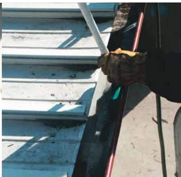
5) Use a soft bristle brush and sweep the dirt out. Rinse again.
