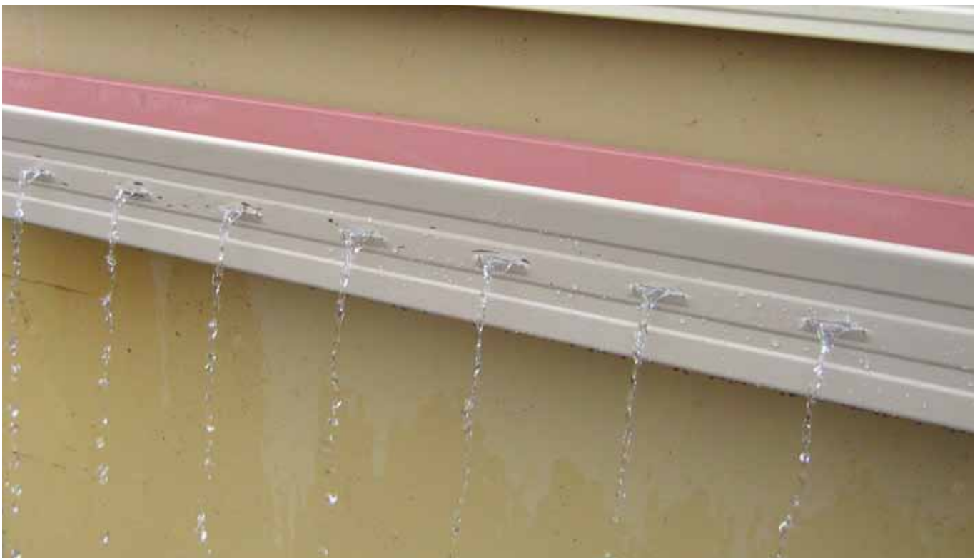
Typical overflow from slotted gutter (gutter shown is not available in all areas.)
